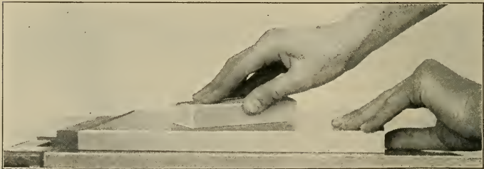
Fig. 120—Sandpapering with Block
